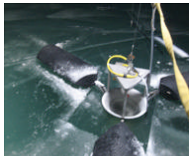
Ice cut out to install a SolarBee mixer
